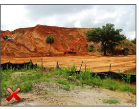
Poorly maintained silt fence surrounding the large stockpile area.
