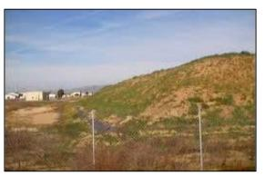
Stockpiles of soil can deliver large amounts of muddy runoff to paved roads, adjacent lawns, and local creeks. A silt fence should be placed around stockpile areas to prevent silt-laden runoff from leaving the site.
