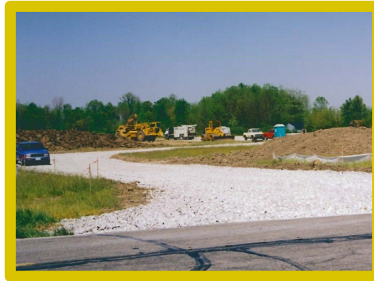
Stone Construction Entrance
