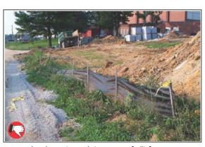
Inadequate maintenance of silt fence.
