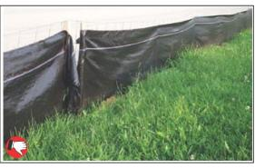
Two sections of silt fence not properly connected. Sections should be overlapped and wrapped together.
