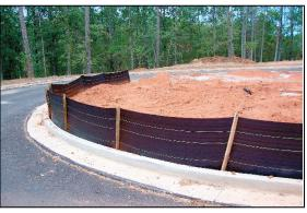
Silt fencing is commonly used to pond, settle, and filter sediment from sheet runoff. On slopes, set back from slope toe to allow for maintenance. Make sure fencing is trenched in properly and stakes are on the downhill side. Inspect frequently to detect and address bypasses, undercutting, and overtopping.
