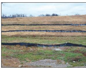
Use multiple sections of silt fence to interrupt long slopes.
