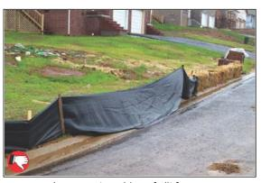
Improper trenching of silt fence.
