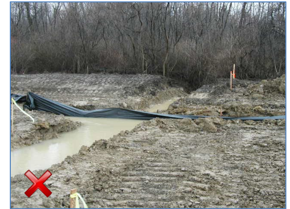
Example of poor sediment trap installation. Silt fencing should never be used as an outlet structure for a sediment trap.
