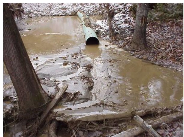
Example of sediment laden illicit discharge from an active construction site. NRCS.
