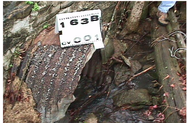
Example of numbering and photographing a stormwater outfall
