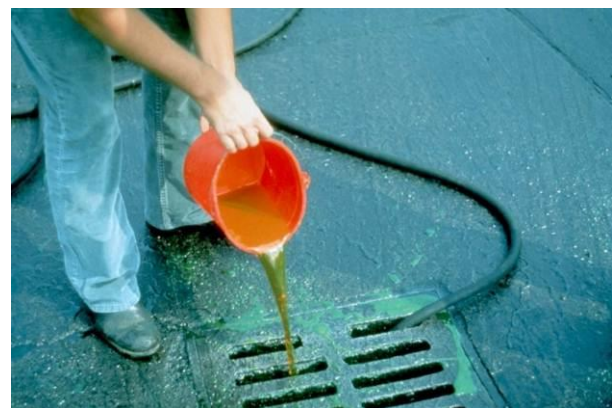
Example of dye testing the stormwater drainage system. Note use of garden hose to flush dye through the system.
