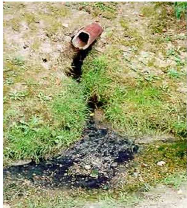
Example of an illicit discharge from a septic system. Stormwater Magazine. October 2003.
