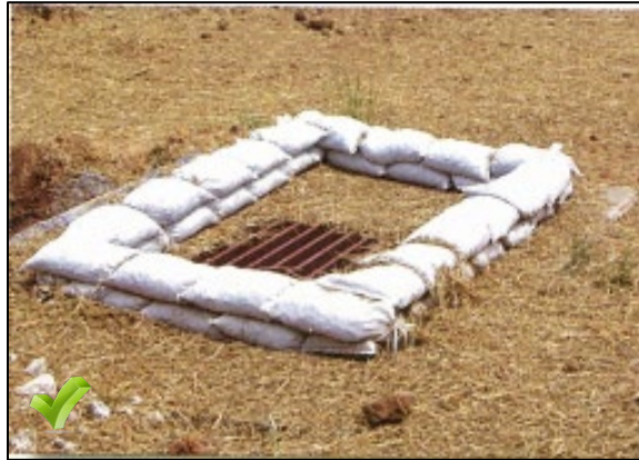
Inlet protection berm construction of half-filled stone bags. Use #57 rock, overlap bags to eliminate large openings and rapid flow-through.
