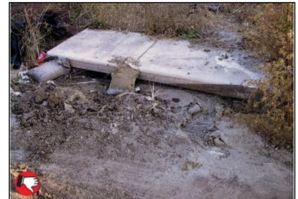
Poor placement and poor maintenance of stone bag inlet ponding dam. Accumulated sediment must be removed and dam should be repaired.
