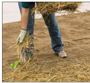
As soon a feasible, sites should be temporarily stabilized with straw, or permanently stabilized with grass and sod. When straw is used, it should be crimped or "punched" into the ground to prevent the straw from moving during wind and rain events. Erosion control mats or sod should be used in concentrated flow areas, such as ditches and swales.
