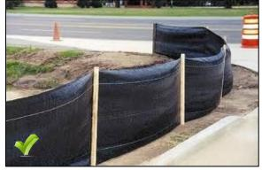
Silt fences should be installed and maintained in disturbed areas to collect sheet flow runoff from the site. Never place a silt fence across concentrated flow, such as a ditch, swale, or drainage channel.
