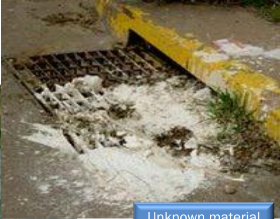
Unknown material dumped on inlet
