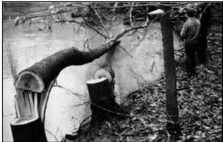
Exhibit 403d: Felled trees anchored to the streambank deflect flows away from the bank to prevent erosion (Source: Ohio Stream Management Guide)
