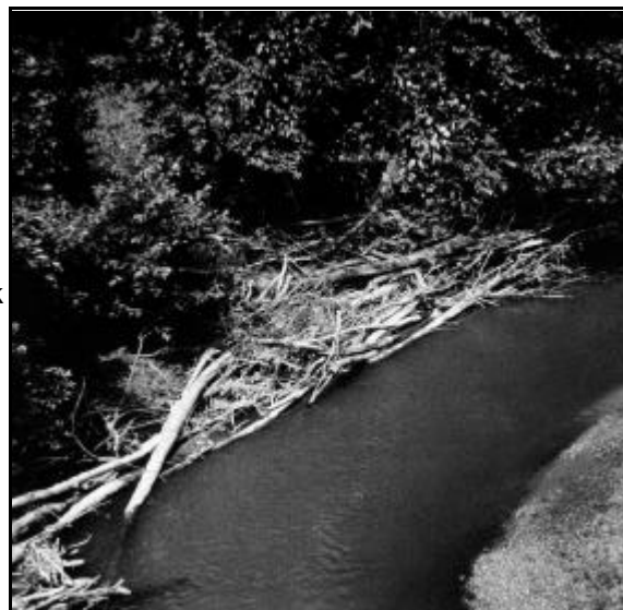
Exhibit 403f: Anchored brush piles are an inexpensive but effective means of bank protection (Source: Ohio Stream Management Guide)
