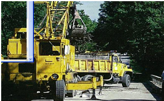
“One-Step Method” for debris jam removal
