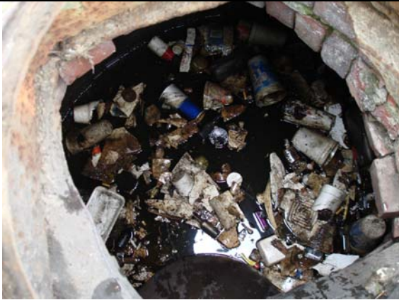
Leaves and other debris can clog storm drains and cause driving hazards.
