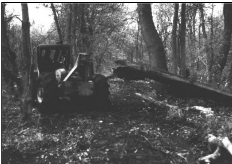
Exhibit 402a: Logjam Removal Using Heavy Machinery (Source: NRCS Files)
