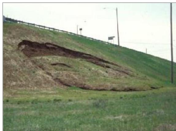
**Figure 13: Example soil failure along embankment**
