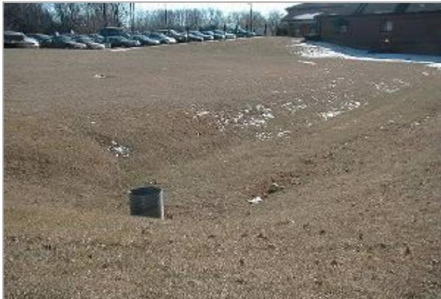
**Figure 3: Example of an infiltration basin**
