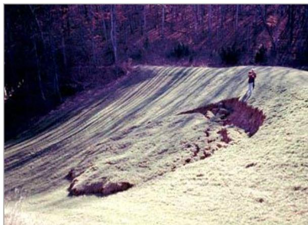
**Figure 18: Soil slump failure of embankment**
