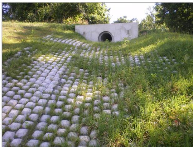
**Figure 19: Armoring of pipe outlet to prevent scour**
