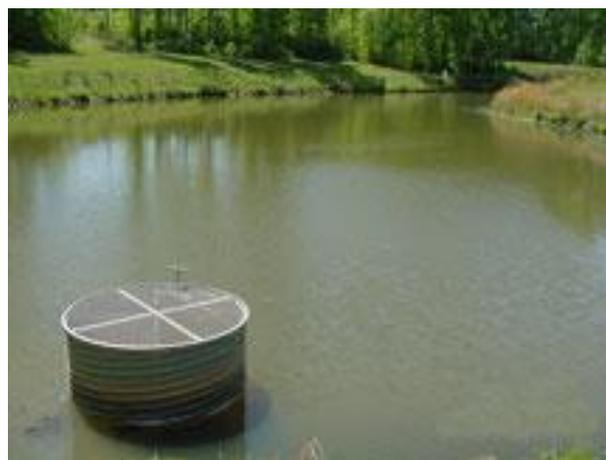
**Figure 2: Example of a wet detention basin**
