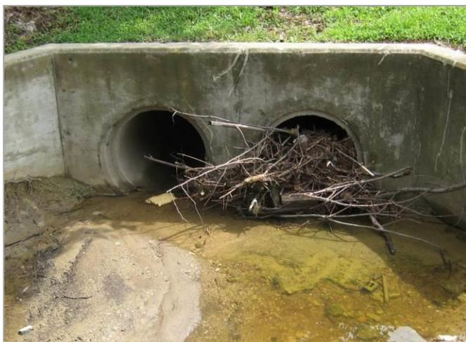
**Figure 16: Blockage caused by inadequate maintenance**
