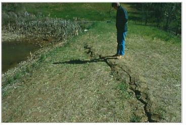
Figure 14: Longitudinal crack along top of embankment
