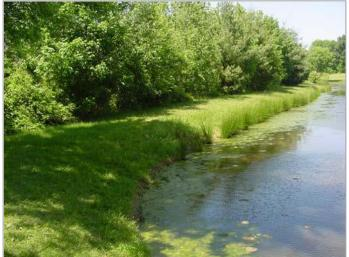
Figure 5: Excessive woody vegetation on dam embankment
