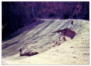
Figure 18: Soil slump failure of embankment
