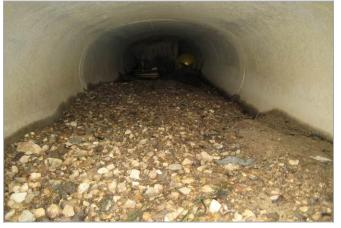
Figure 8: Sediment / debris accumulation in pipe
