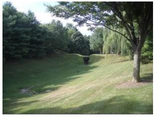
Figure 1: Example of a dry detention basin
