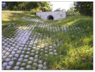
Figure 19: Armoring of pipe outlet to prevent scour
