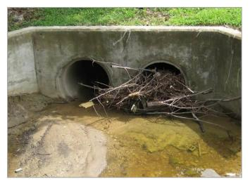
Figure 16: Blockage caused by inadequate maintenance
