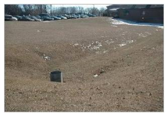
Figure 3: Example of an infiltration basin
