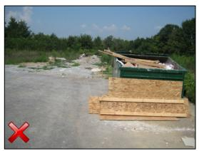
Large pieces of construction waste should be broken down and placed inside the designated disposal dumpster. Material piled up in the background should also be placed in the dumpster.
