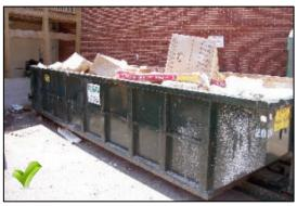
Majority of the construction waste is contained inside the dumpster. Liquids should never be emptied in the dumpster.
