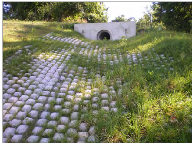
Figure 19: Armoring of pipe outlet to prevent scour
