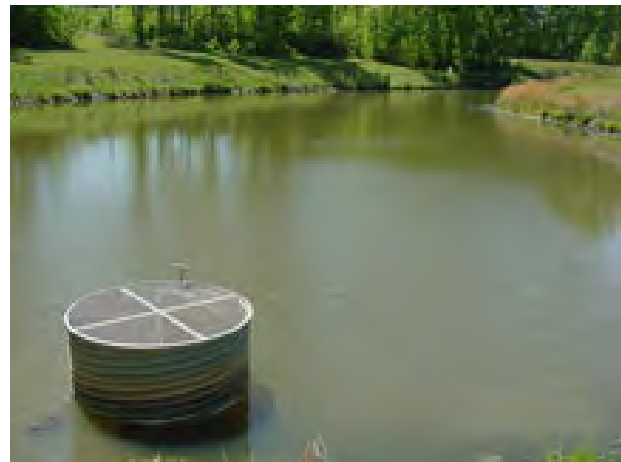
Figure 2: Example of a wet detention basin
