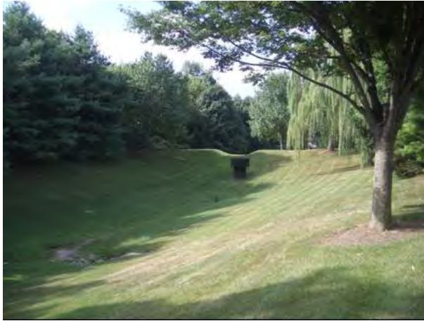
Figure 1: Example of a dry detention basin
