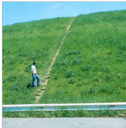
Figure 22: Regular pedestrian traffic
