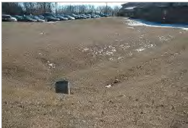
Figure 3: Example of an infiltration basin
