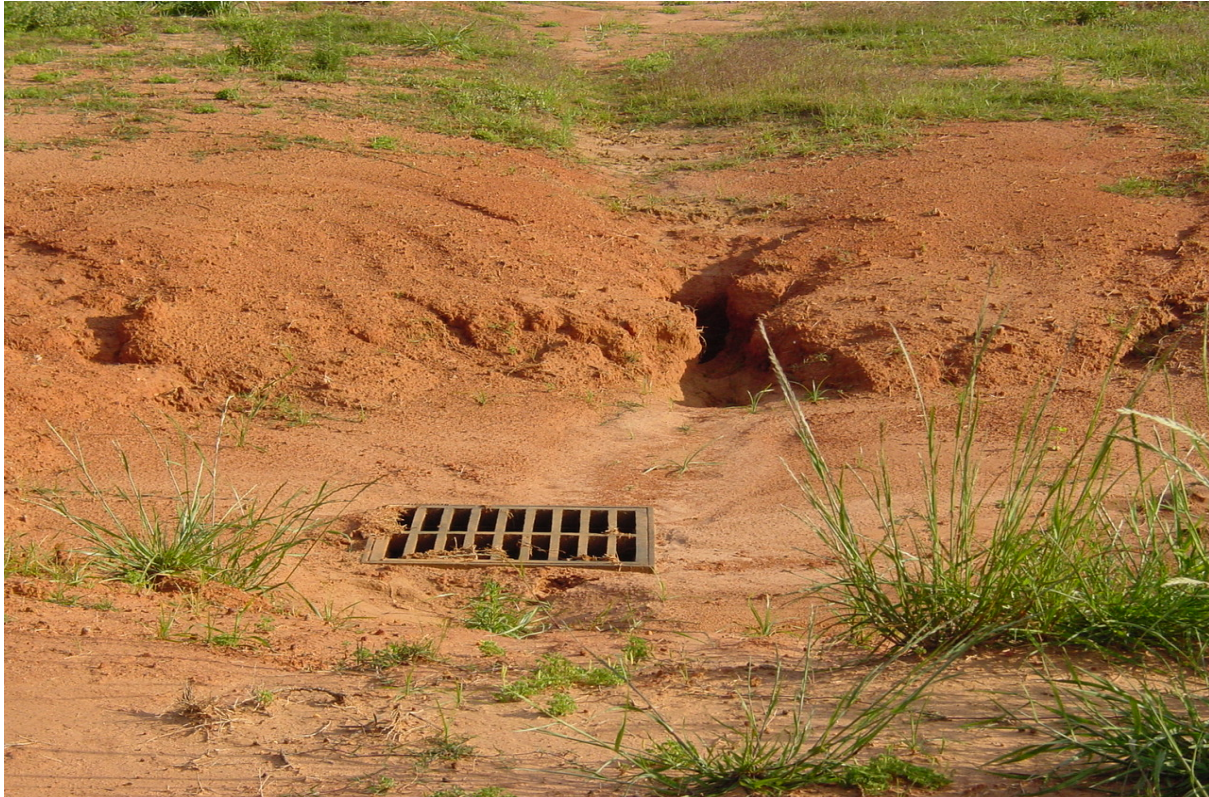
Figure 3.2. Rill and Gully Erosion
